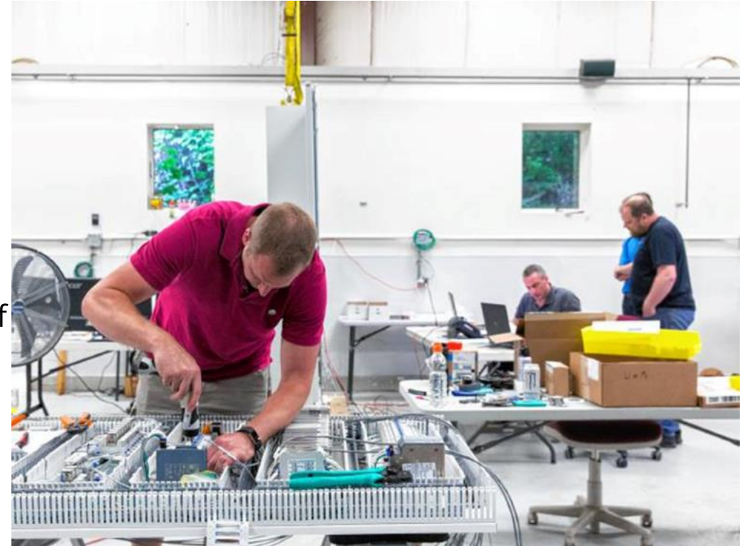
Ewing Controls – converted 2017
